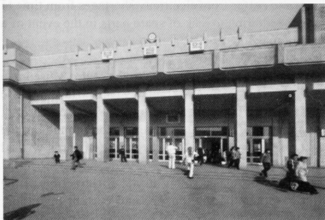
Puhung station entrance. Photo John Smiles
